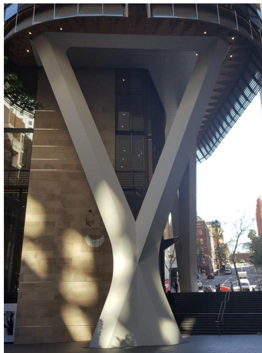
Figure 1. Concrete filled steel column, 200 George Street, Sydney
