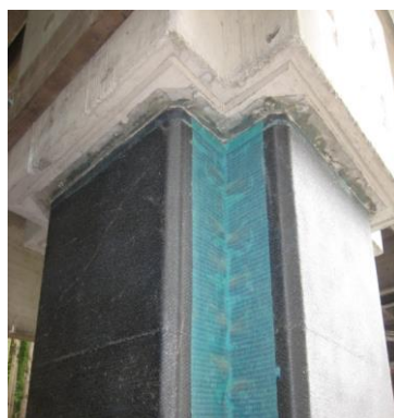
(c) Column confinement (Non-conventional)
