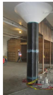
(b) Column confinement (Conventional)
